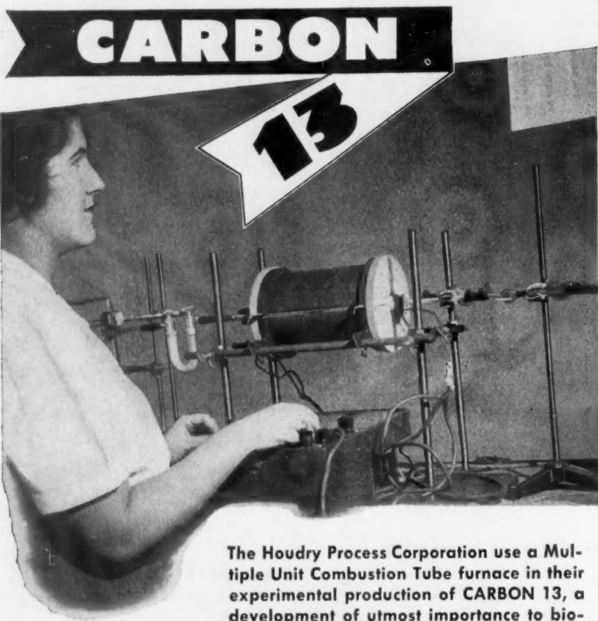
A Multiple Unit Combustion Tube Furnace in operation at The Houdry Process Corporation, Philadelphia.
